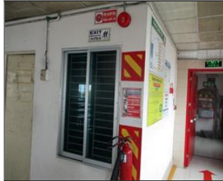
Photo of fire safety equipment Fire safety to confirm the sustenance-Fire alarm.JPG
