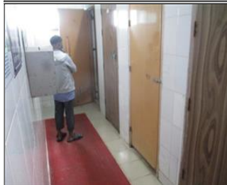
Photo of the sanitary facilities Hygiene sensitive area-Toilet.JPG
