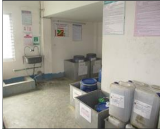
Photo of chemical storage room (if applicable) High risk area-chemical store.JPG
