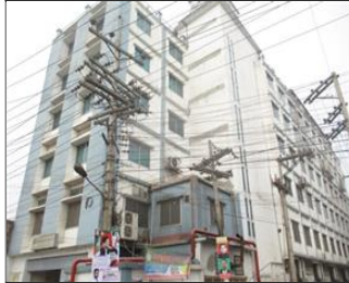
External photo(s) of the production unit(s) Facility outlook.JPG
